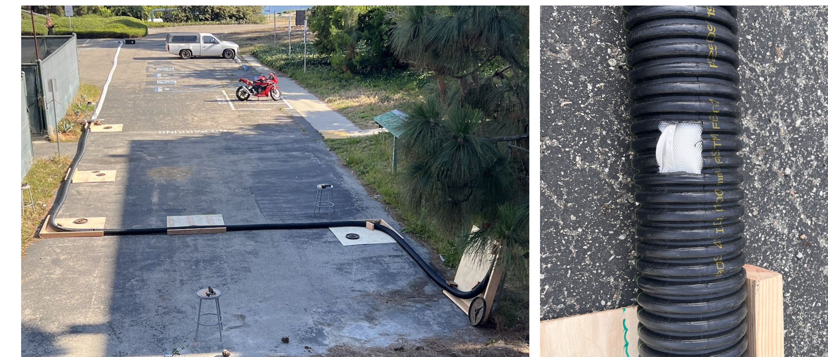
Figure 5, 6: Conduit Track Setup, Deployed Cables.
