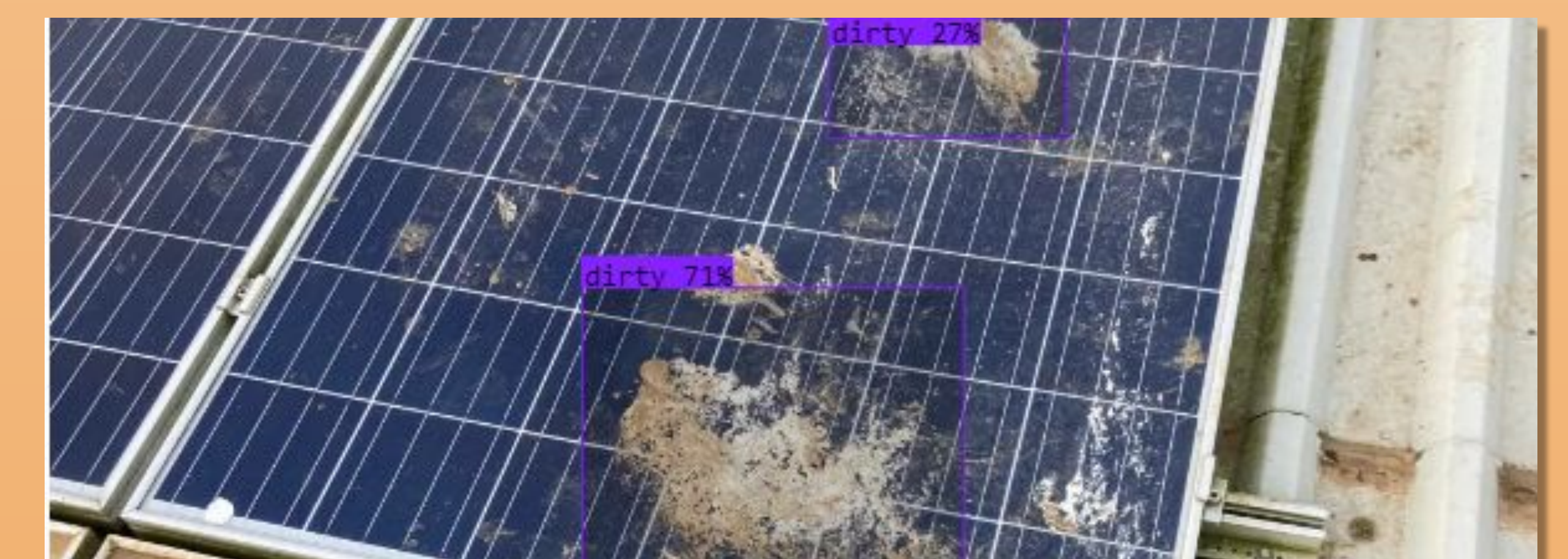
Simulated output of live filtering on RGB image finding dirt
